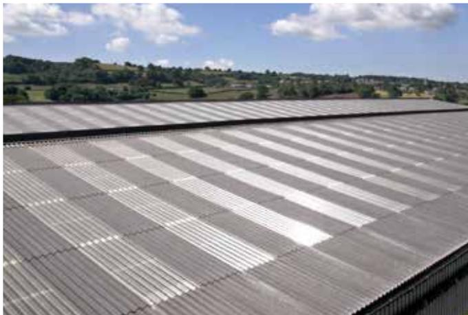
Site assembled (built-up) rooflights are supplied as translucent sheet profiled to match both the weather sheet and liner panels, with a separate intermediate layer for thermal performance.
