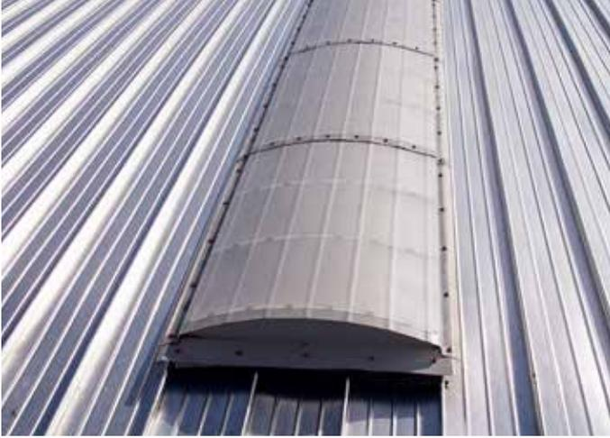
A number of proprietary barrel-vault systems are available. They are usually specified with Secret Fix Systems and for very low pitches. They can be used with single skin, built-up or composite roofs, with secret fix systems, curved roofs, flat roofs, along a ridge and in other low pitch applications.
