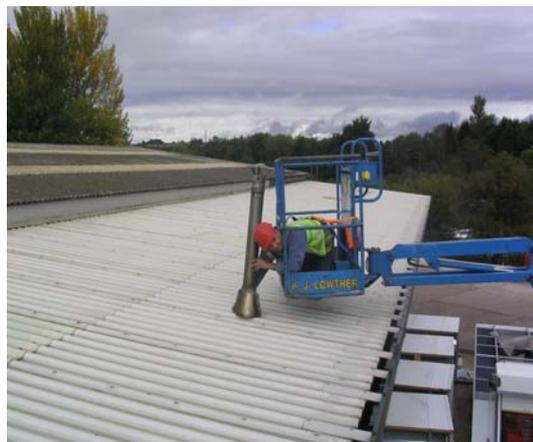
**Figure 3 Using a MEWP to inspect a vent**
