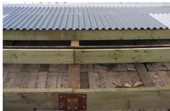
**Figure 7 A crash deck providing collective fall protection**
