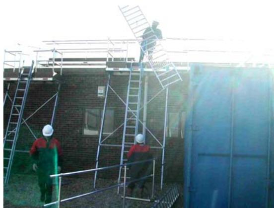
**Figure 4 Installing a proprietary edge protection system**
