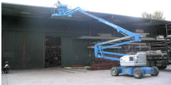
**Figure 5 Using a MEWP to clean the gutter**
