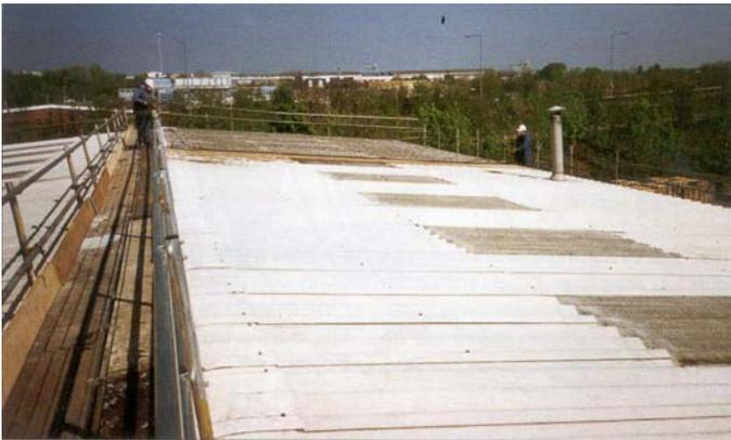
**Figure 12 Complete overlidding of an AC roof**
