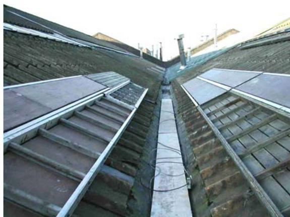
**Figure 6 A partially boarded out valley gutter (another line of boards needed to reach 2<sup>nd</sup> purlin line)**
